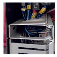
The cable trays used to carry electrical installations in control and switchgear cabinets.
