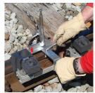
• Used to remove the slag from the crucible area of the mold after making a nVent ERICO Cadweld connection
